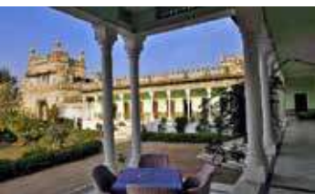
20th c. The Piramal Haveli, Rajasthan (Marwari)
